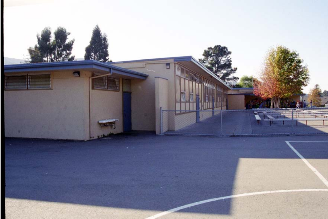
Figure 5: North Face of Main Building
