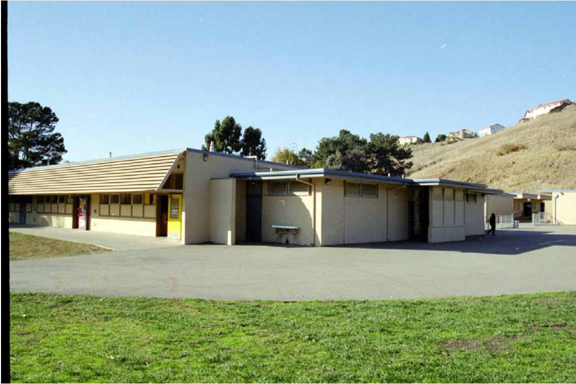
Figure 4: Southeast Corner of Main Building
