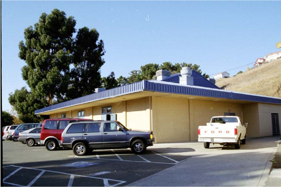
Figure 11: South Corner of Multi-Purpose Building
