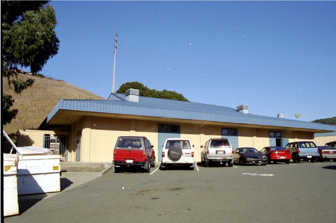
Figure 12: South Face of Multi-Purpose Building
