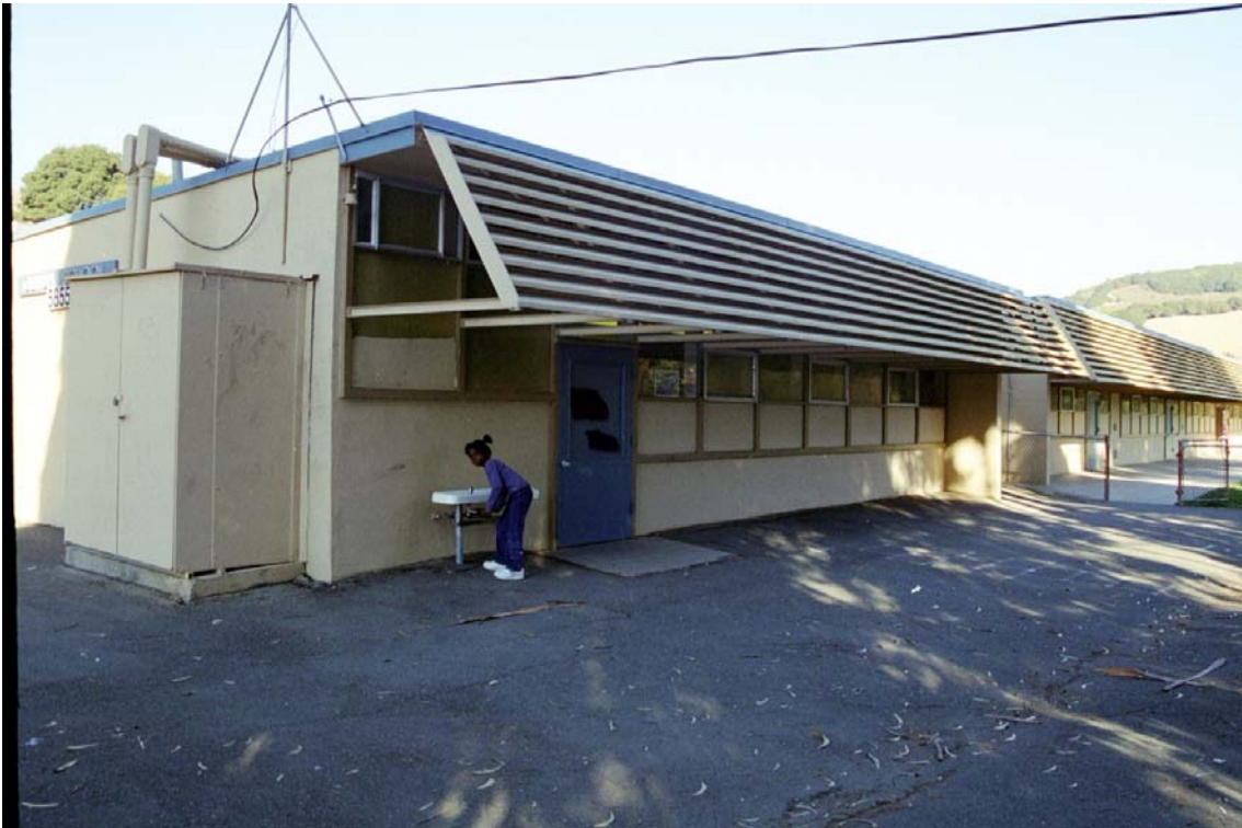
Figure 3: South Face of Main Building
