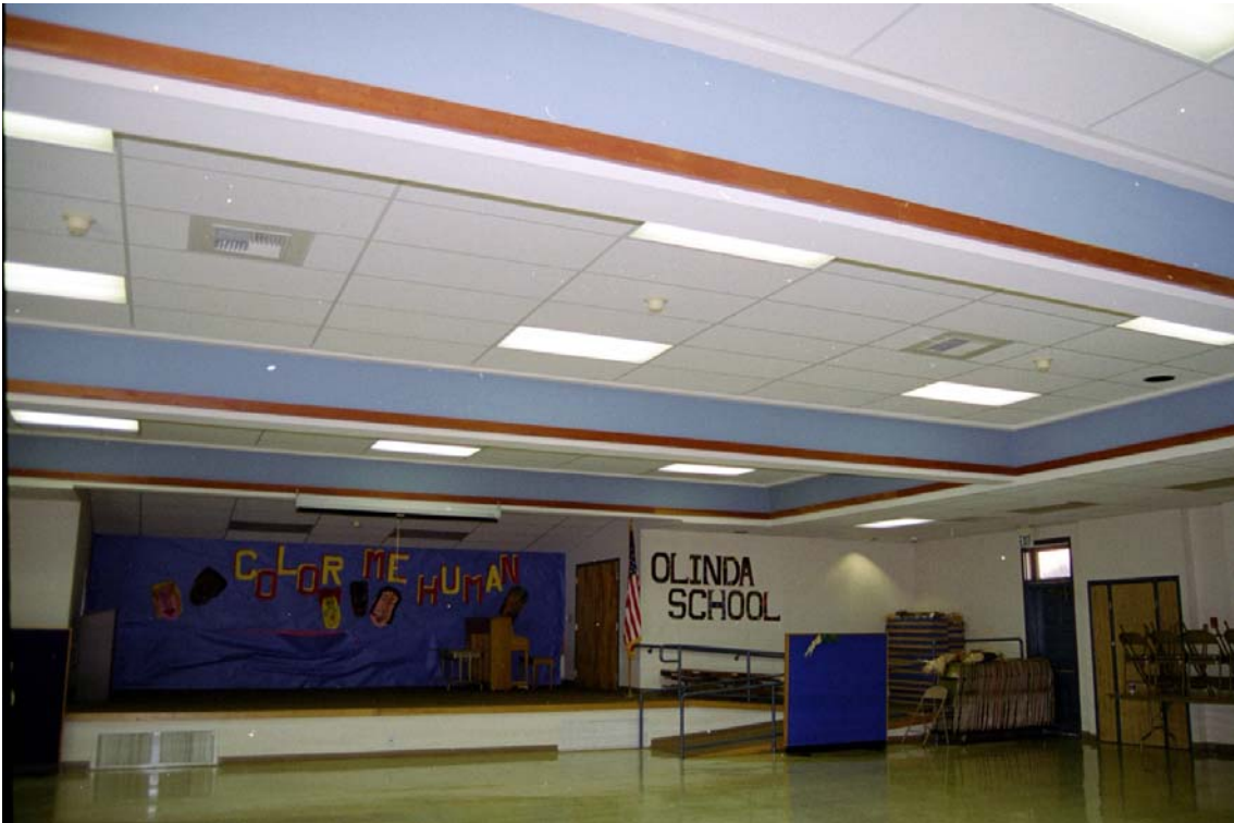
Figure 13: Interior of Multi-Purpose Building
