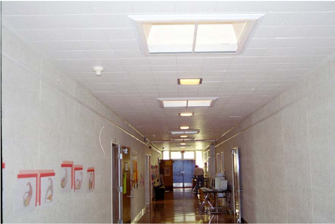
Figure 9: Central Longitudinal Corridor of Main Building
