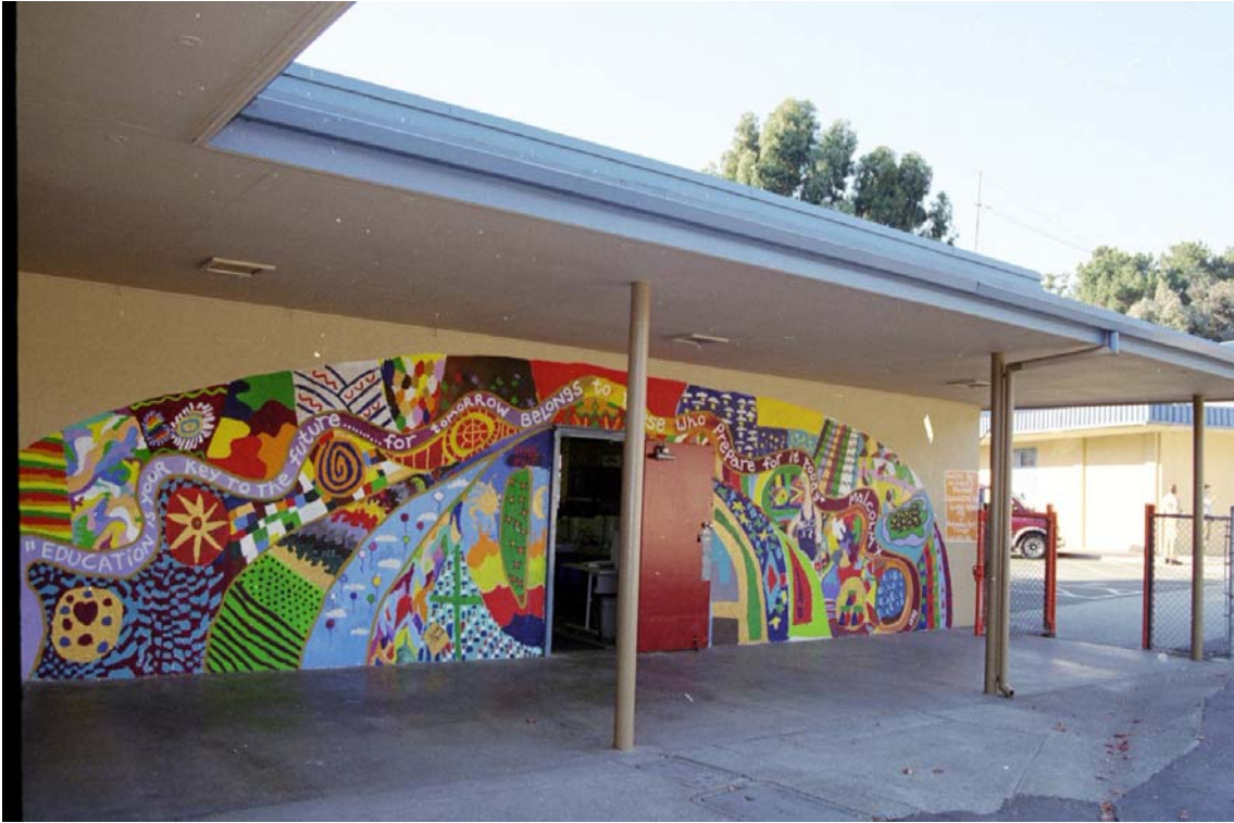
Figure 7: East Face of Computer Room Wing of Main Building
