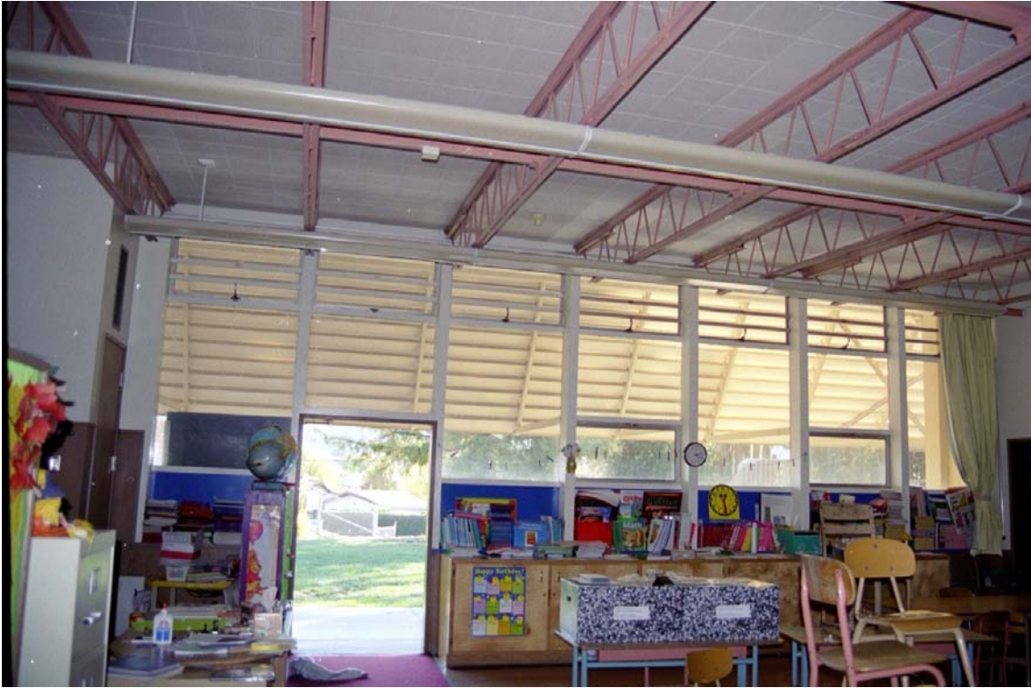
Figure 10: Typical Classroom Interior at Main Building
