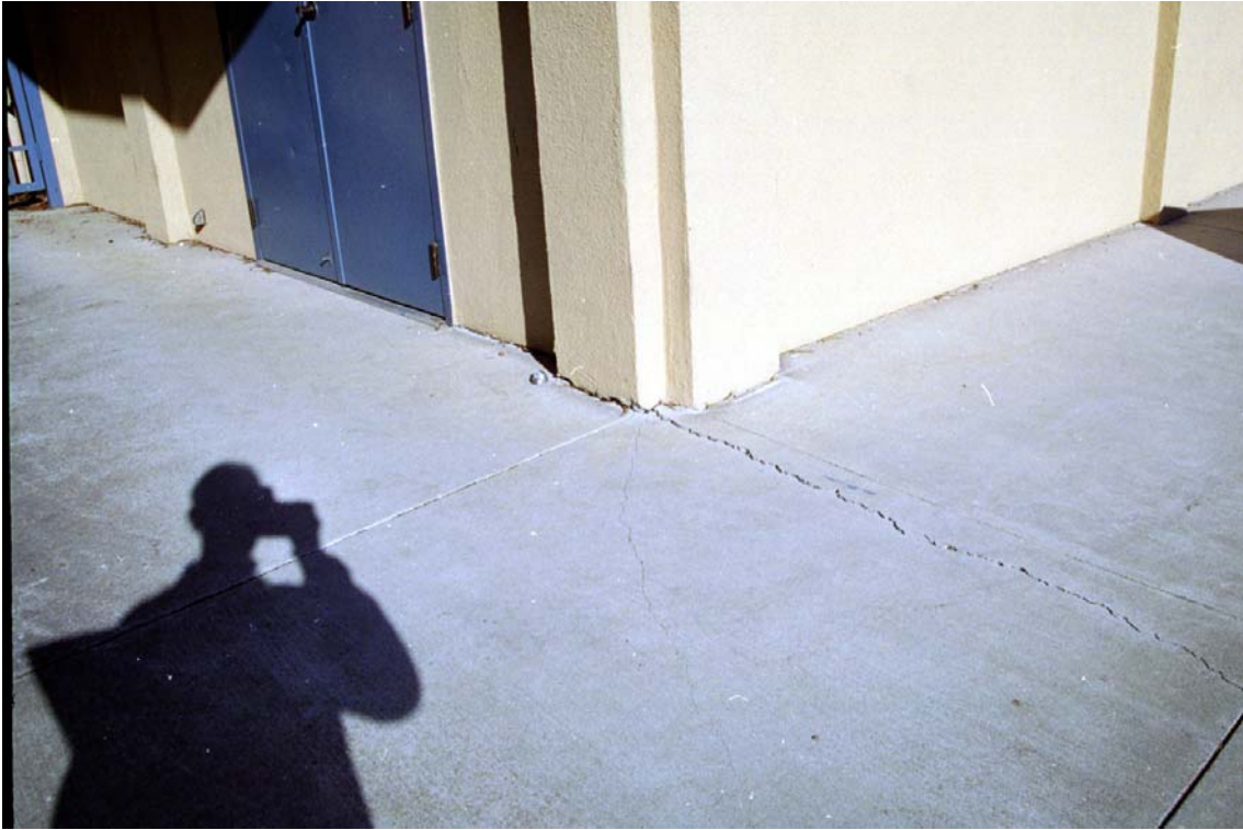
Figure 14: Cracks in Exterior Slab at Main Building
