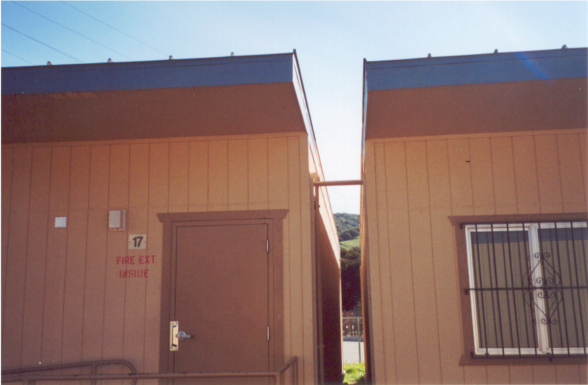
Figure 16: Conduit Running between Portable Units
