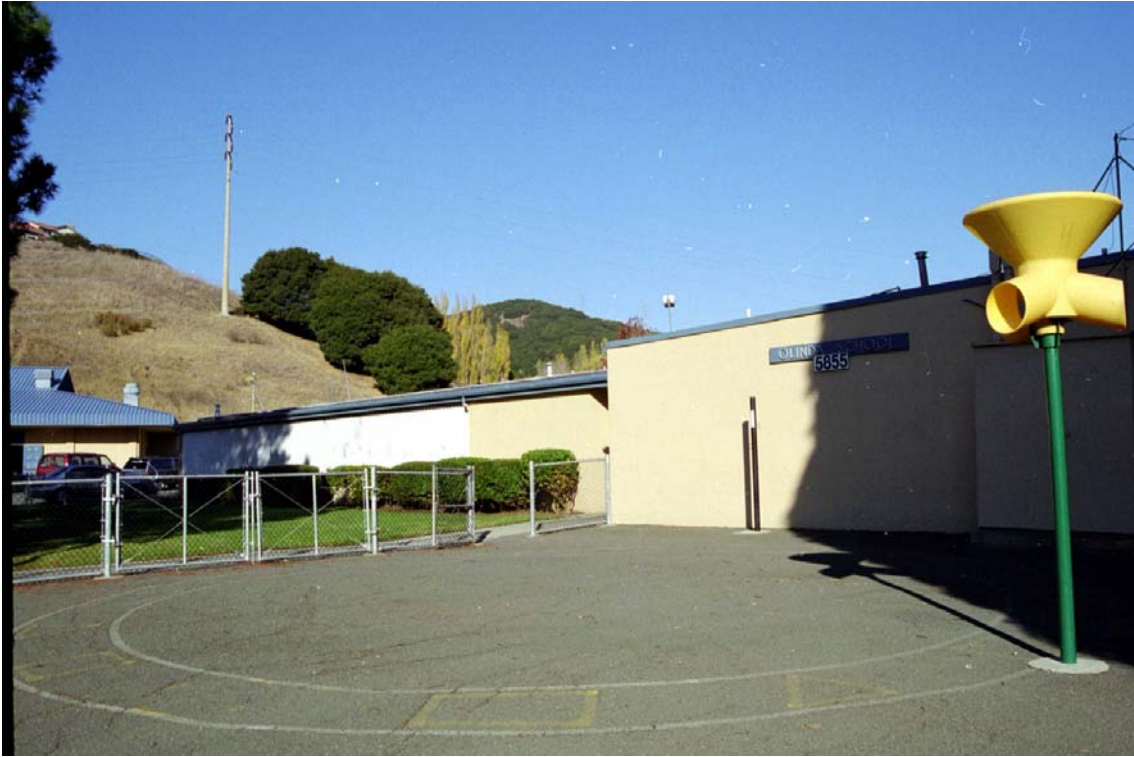
Figure 2: West Face of Main Building
