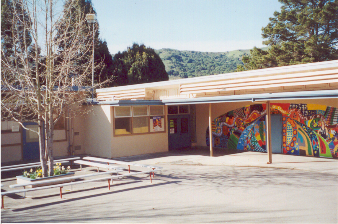
Figure 6: Re-entrant Corner at Main Building
