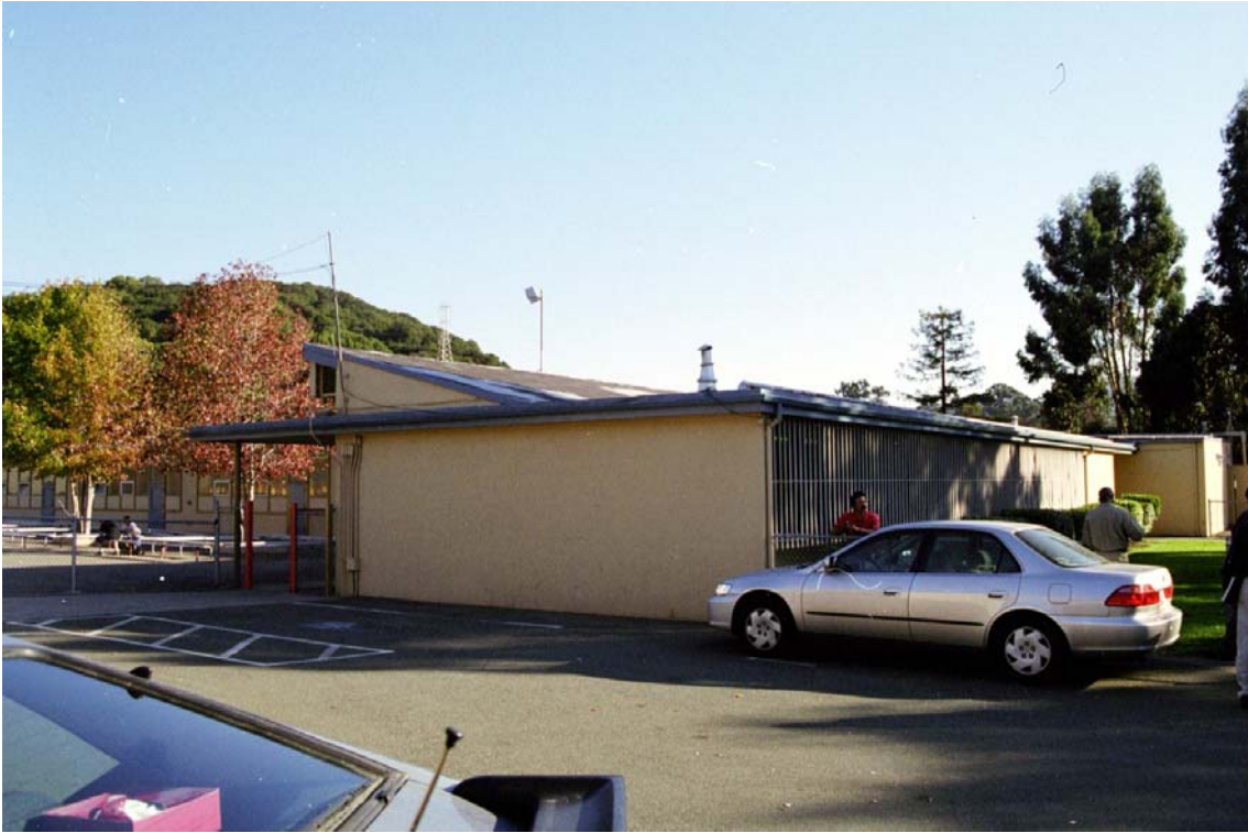
Figure 8: Northwest Corner of Main Building
